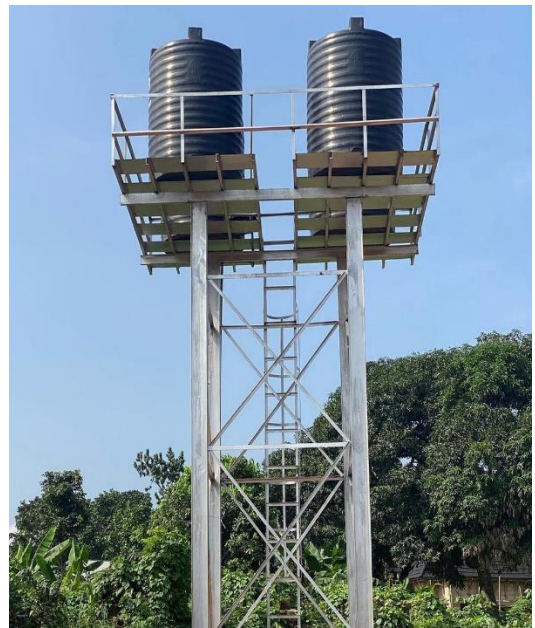
FIG 1.3 WATER STORAGE TANK STAND BEFORE COMPLETION AND AFTER
