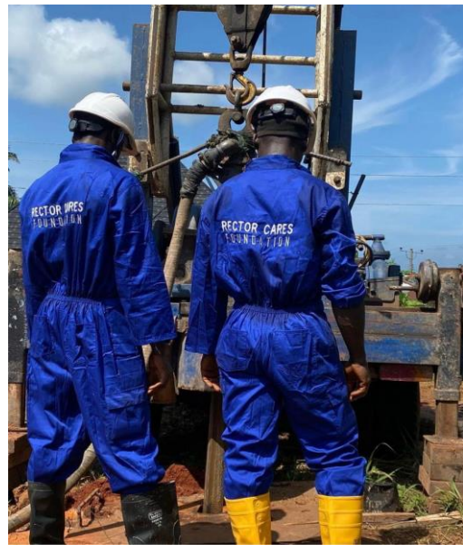
FIG 1.1 DRILLING MACHINE USED TO DRILL 350 FT BELOW GROUND LEVEL
